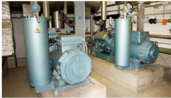
**Figure 9: High temperature heat pump at Mohrenbrauerei in Dornbirn (Klima:aktiv, 2012)**
