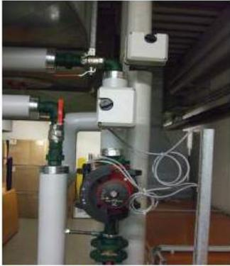
**Figure 18: high efficient pump (klima:aktiv, 2012c)**
