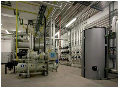
**Figure 15: compression heat pump at Daily Service Tiefkühllogistik GesmbH & Co KG (Klima:aktiv, 2012b)**
