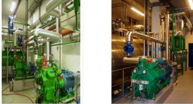
**Figure 11: Pictures of two “hybrid” heat pumps by “Hybrid Energy AS”left: 300 kW, right: 650 kW heating capacity (Nordtvedt, 2009)**
