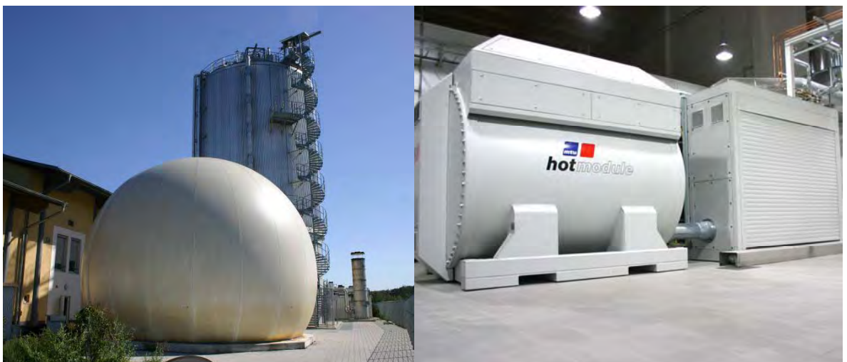
Figure 4.40 Biogas plant in Leonberg, Germany and Fuel Cell, HotModule, MTU Onsite Energy (Source: MTU Onsite Energy, Germany)
